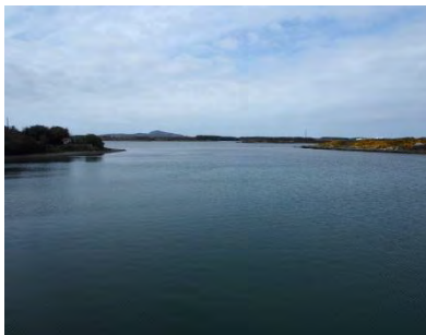
View north from Four Mile Bridge, showing lagoon between embankments.
